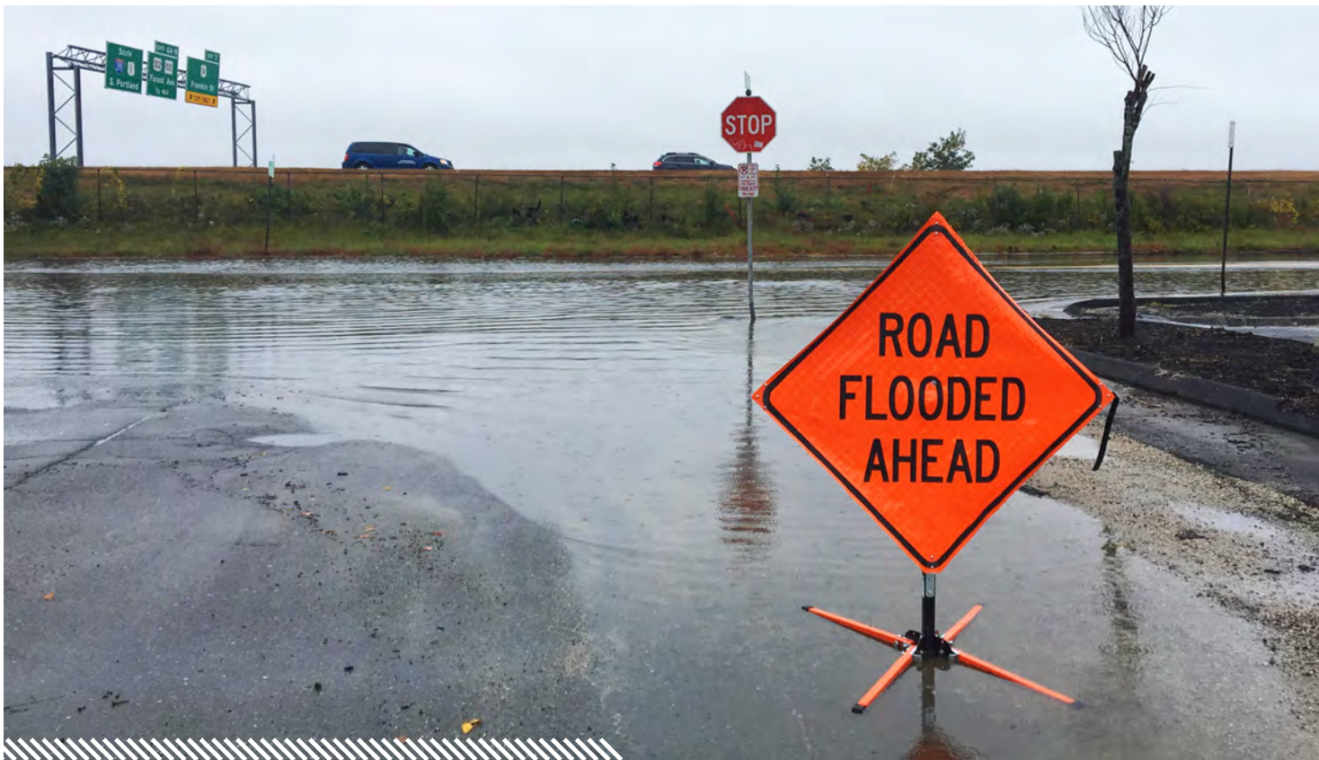
HIGH TIDE FLOODING, MARGINAL WAY • Photo by Ian Johnson
