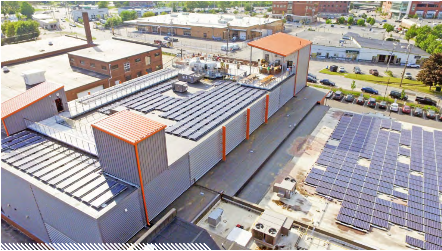
SOLAR ON BAYSIDE BOWL • Photo by ReVision Energy
