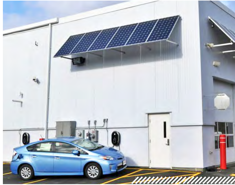
ELECTRIC VEHICLE CHARGING WITH SOLAR POWER • Photo by ReVision Energy
